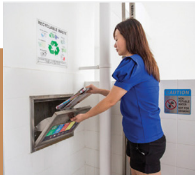
SEPARATE CHUTES FOR RECYCLABLE WASTE
