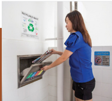
SEPARATE CHUTES FOR RECYCLABLE WASTE
