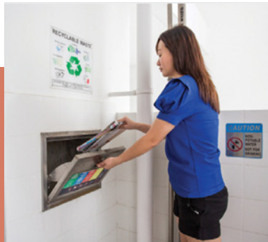
SEPARATE CHUTES FOR RECYCLABLE WASTE
