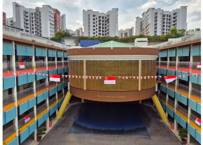
Photo courtesy of Temasek Primary School
